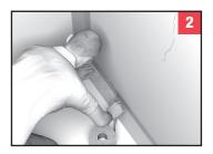
Bed a strip of membrane tape into the coating while still wet to strengthen and reinforce the junction points.
