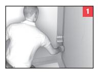
Apply coating to the junctions between wall to floor and wall to wall corners using a paint brush or short pile roller at coverage 0.5kg/sqm.
