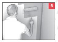
When dry, apply a uniform coating over the complete wall and floor area in a continuous layer at a coverage of 0.5kg/sqm using a paint brush or roller as previous. Allow to dry for 2 hours before applying a second coat to the same area at the same at coverage 0.5kg/sqm. Allow 24-48 hours drying before commencing tiling.
