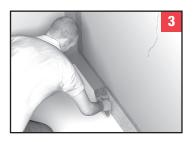
Immediately apply a further application of the coating to the bedded tape to encapsulate at coverage 0.5kg/sqm. Allow to dry for 2 hours.
