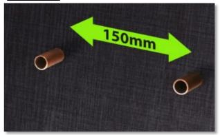
Drill **15mm** holes with the hole centres **150mm** apart and feed copper pipe work through.
