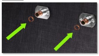
3 Slide the **copper olives** over the pipes until they touch the brackets.
