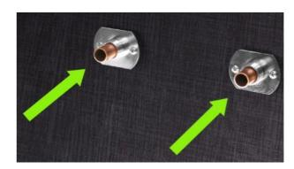
2 Slide the **Brackets** over the pipes and mark drill holes.
